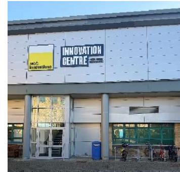
Exterior view of the NOC
