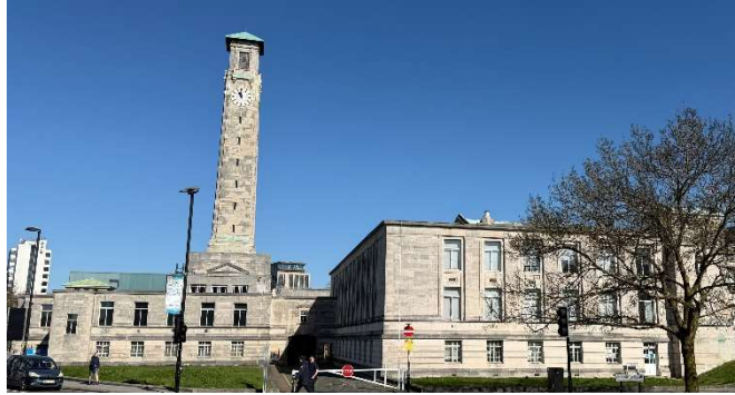
Exterior view of the SeaCity Museum in Southampton
